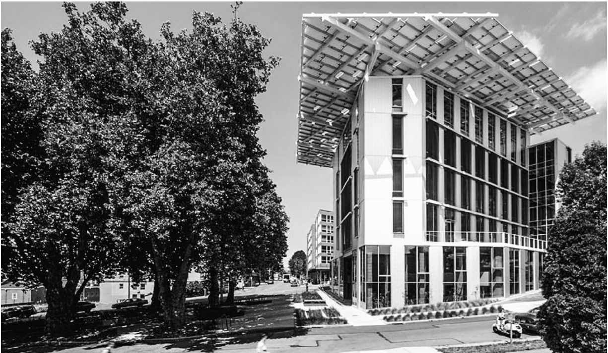
The Bullitt Center in Seattle is one of the greenest commercial buildings in the world.
